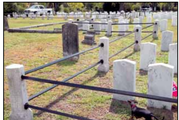
As part of the Fence Restoration Project, two-level steel rail fence which borders the 700-plus buried Confederate soldiers in the Gettysburg section of Laurel Grove Cemetery, Savannah, GA and adjacent areas has been thoroughly smoothed, primed and then painted by members of the Savannah Militia Camp 1657 , Savannah, GA.
