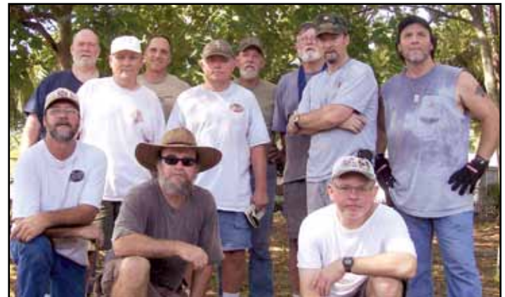
Kirby-Smith Camp 1209 , Jacksonville, FL, held a dual-cemetery workday. Members began the day at Old City Cemetery, where a large tree was removed that was crumbling a portion of the brick wall which surrounds the cemetery. Next it was on to Camp Captain Mooney Cemetery, where general cleanup was done. Camp Captain Mooney Cemetery is thought to be the site of a skirmish in 1864, in which seven Confederate soldiers were killed and buried where they fell.
