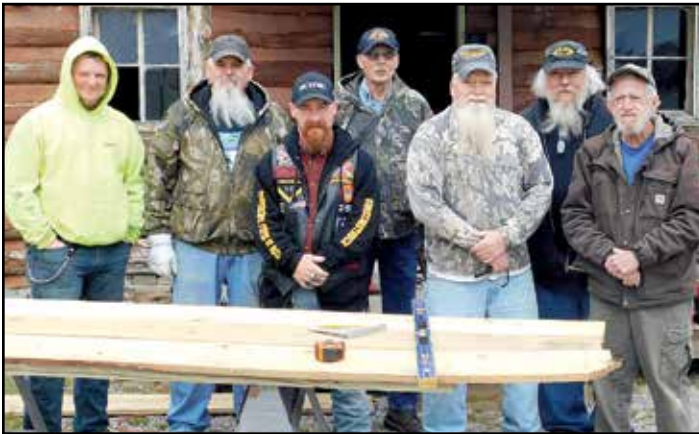
General Lloyd Tilghman Camp 1495 , Paducah KY, members work on their little log cabin at Arant's Confederate Park, with help from SCV brothers from Forrest's Orphans Camp 1744 , Calhoun, KY.
