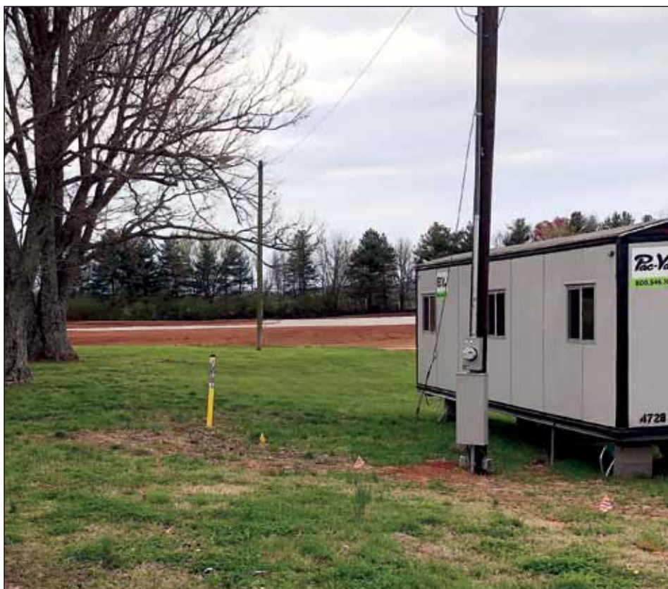
A view in March, 2018 of the construction site of the new SCV Confederate Museum at Elm Springs.
