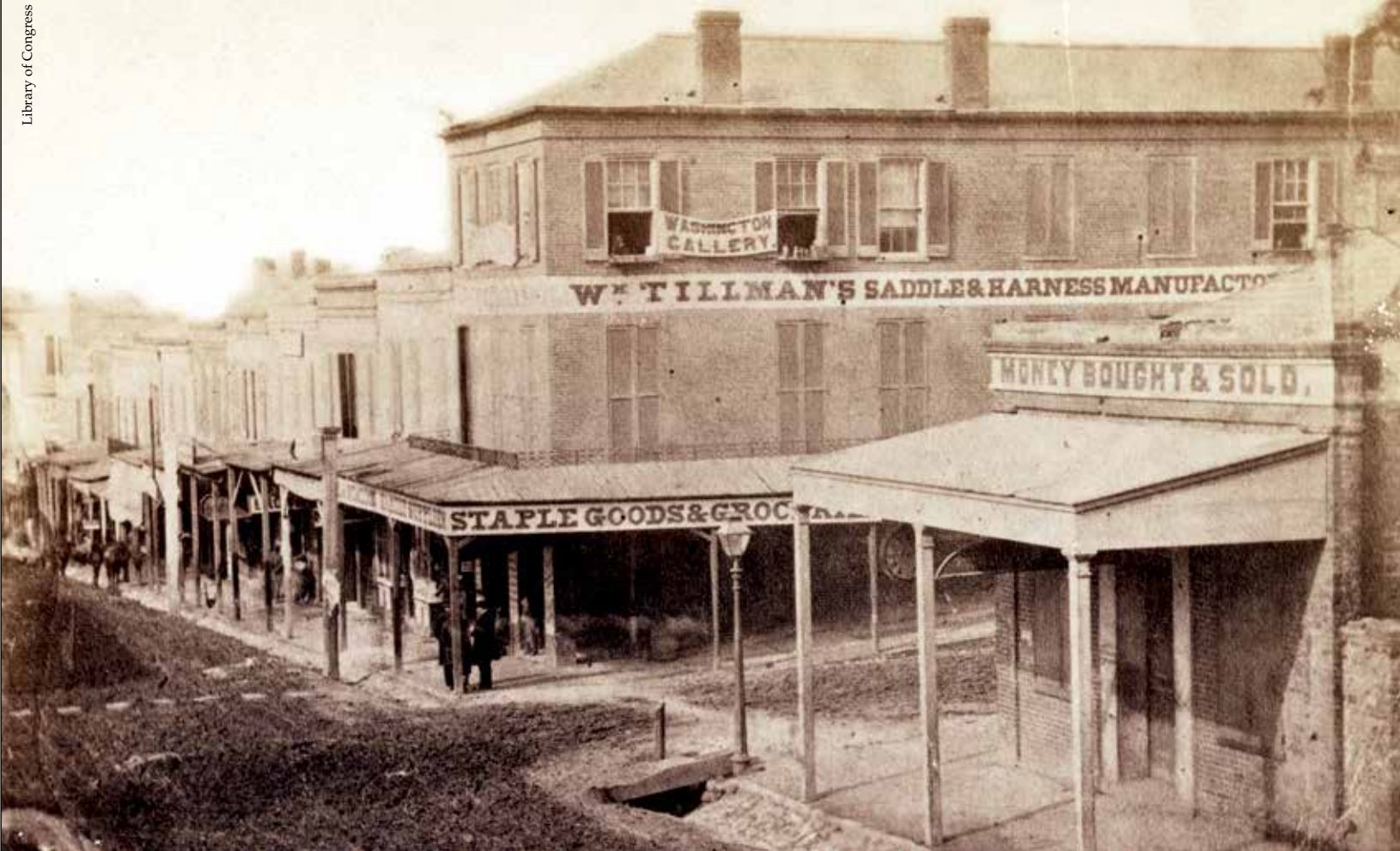
The corner of Washington and Clay Streets, Vicksburg. This is still one of the most prominent intersections in the city.
