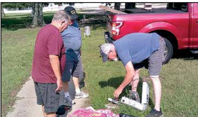
Sam Davis Camp 596 , Biloxi, MS, members, Mike Carter, Ken Overstreet, Rick Randazzo, Don McFall and Joe Newman repaired and re-mounted electric outlet 6 at Beauvoir's camper parking area.
